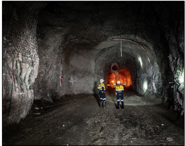
Figure 2: Mt Mann Underground
