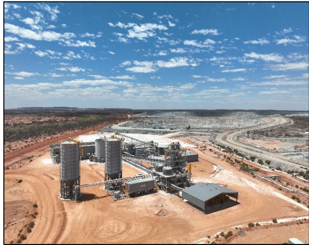
Figure 4: 4Mtpa Paste Plant
