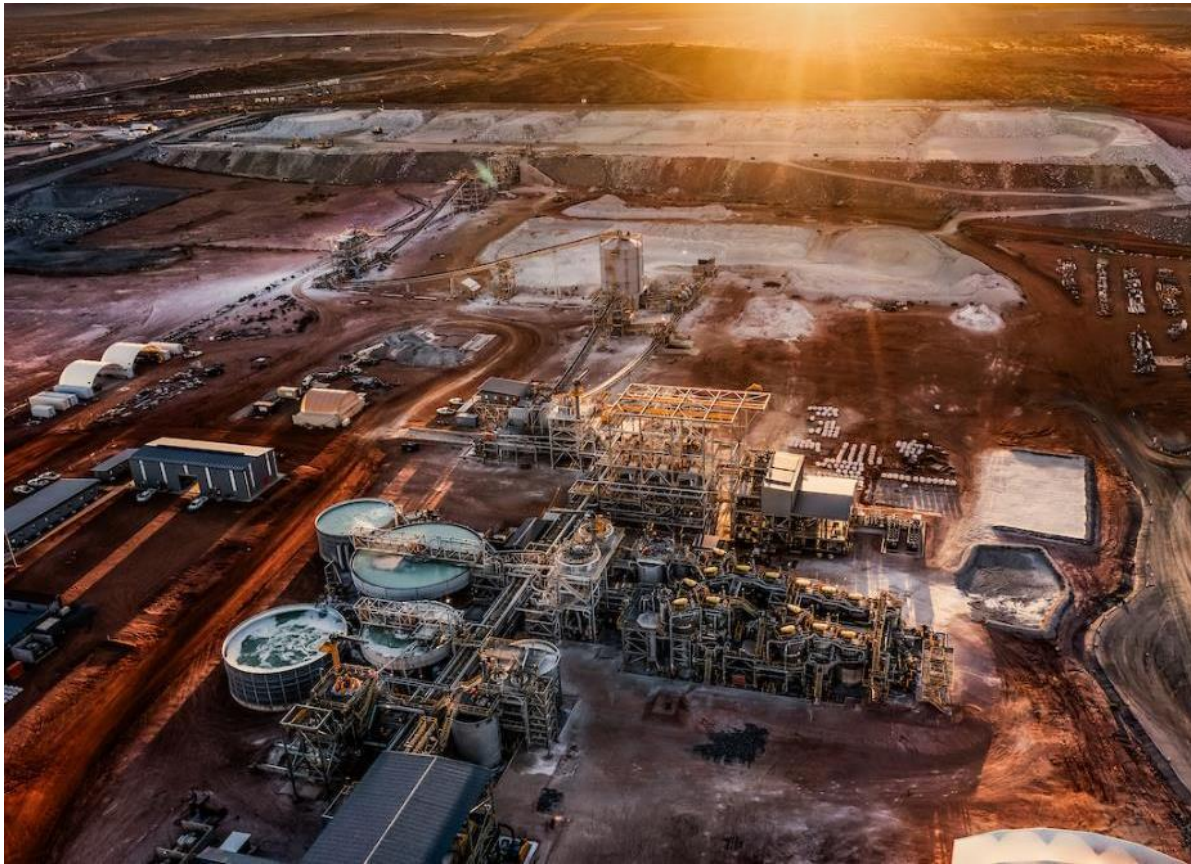
Aerial view of Kathleen Valley process plant
