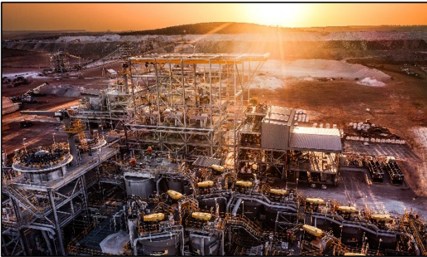
Figure 4: Aerial view of the process plant
