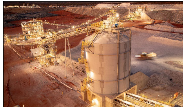
Figure 7: Aerial view of crusher circuit and fine ore bin
