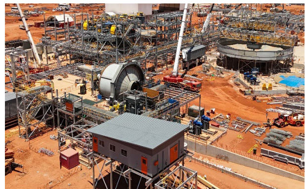
Figure 14: SAG mill and magnetic separation steelwork
