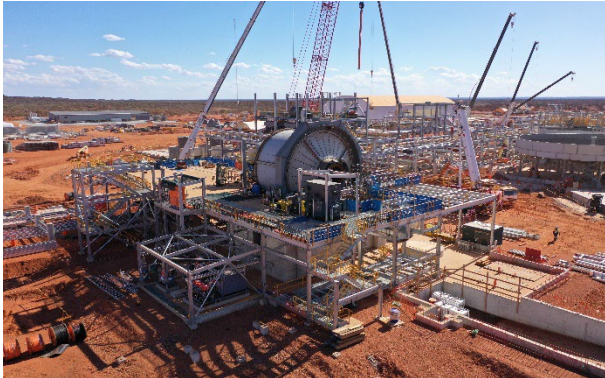
Figure 15: SAG Mill and grinding area steel work
