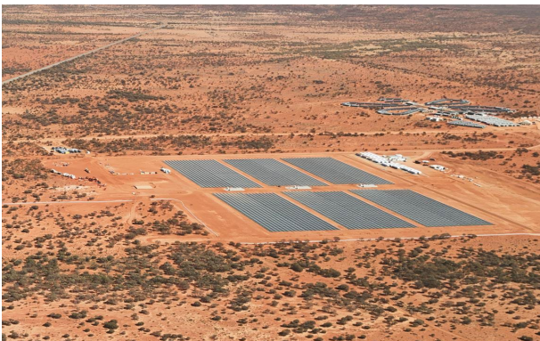
Figure 21: Installation of 31,000 solar panels completed
