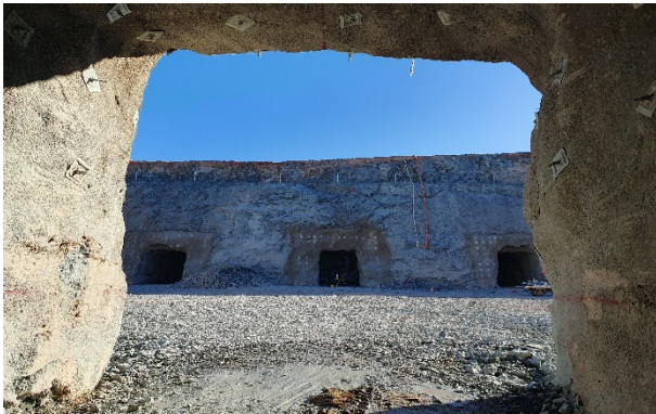
Figure 5: Ground level view looking towards access portals
