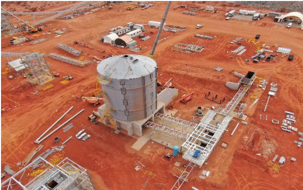
Figure 11: Fine ore bin roof was installed subsequent to the quarter
