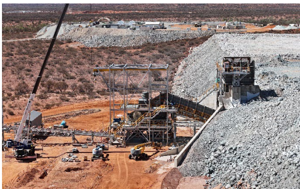
Figure 13: Primary crusher and ROM pad in background
