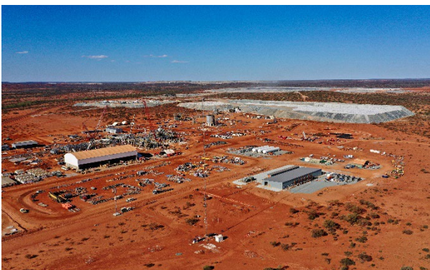
Figure 9: Kathleen Valley site view looking north-east
