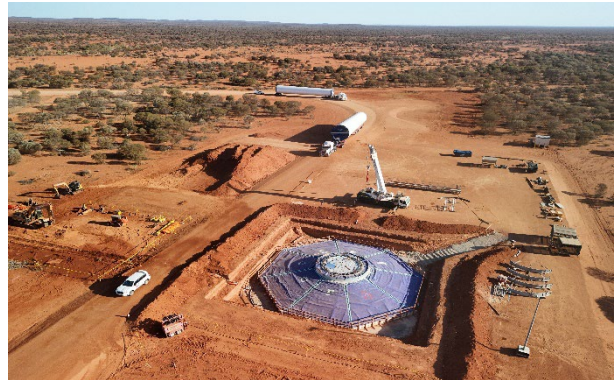
Figure 18: Foundations for wind turbines
