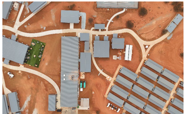
Figure 26: Wet mess and convenience shop officially opened
