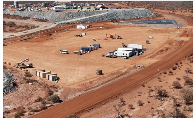
Figure 12: Pastefill plant, earthworks and contractor facilities
