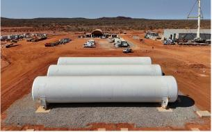
Figure 16: LNG storage vessels
