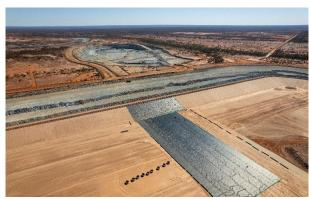
Figure 6: TSF lining in progress
