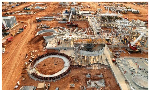
Figure 8: Process Plant concrete nearing completion
