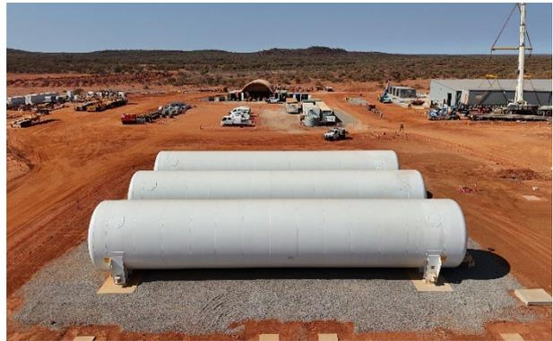
Figure 16: LNG storage vessels
