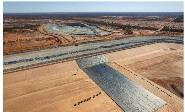
Figure 6: TSF lining in progress
