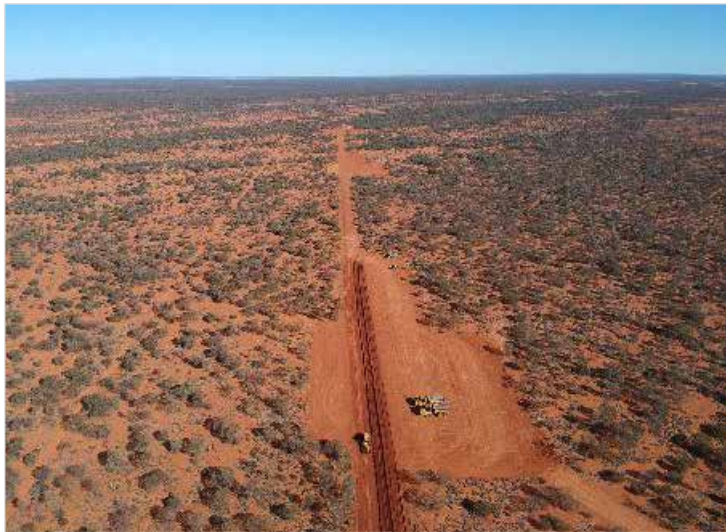
Minimised footprint at the wind turbine farm
