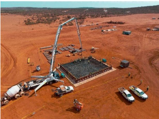
Figure 1: Pouring of the concrete foundation for the SAG Mill
