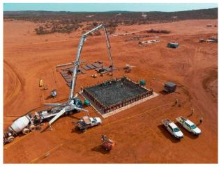
Figure 1: Pouring of the concrete foundation for the SAG Mill
